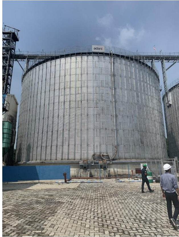
Figure 13: Steel Silo – Junheta, Hoshangabad
